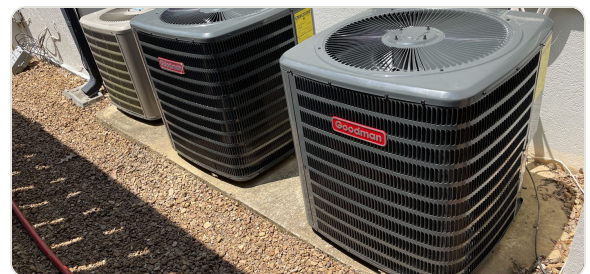
still captured from a walkthrough · two Goodman condensers and a third, older unit.
